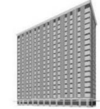
BROCK COMMONS TALLWOOD HOUSE Vancouver, Canada 18 stories | 2017
